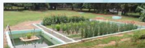
Constructed wetland for waste water treatment
